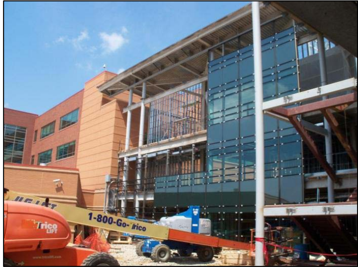
Figure 16 - View of west elevation curtain wall system under construction. The boom lift used during construction of the façade system can be seen at the bottom of the photo. Personal photograph taken by Chris Pozza.
