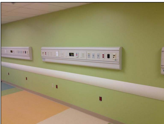
Figure 62 - Modular headwall units used on the project. This image was taken on the third floor of the KP Medical Office Building. Personal photograph taken by Chris Pozza.
