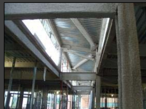
Clerestory spanning 3 rd floor addition.
