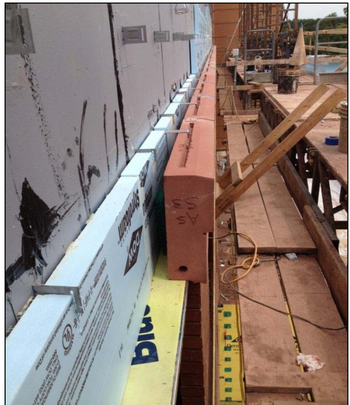
Figure 10 - Precast concrete can be seen above which make up the accent band along with east elevation. Personal photograph taken by Chris Pozza.
