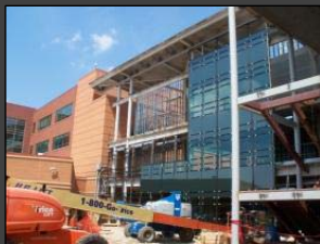
West Elevation Glass Curtain Wall.
