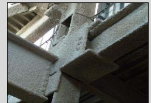
Column-to-beam moment connection.
