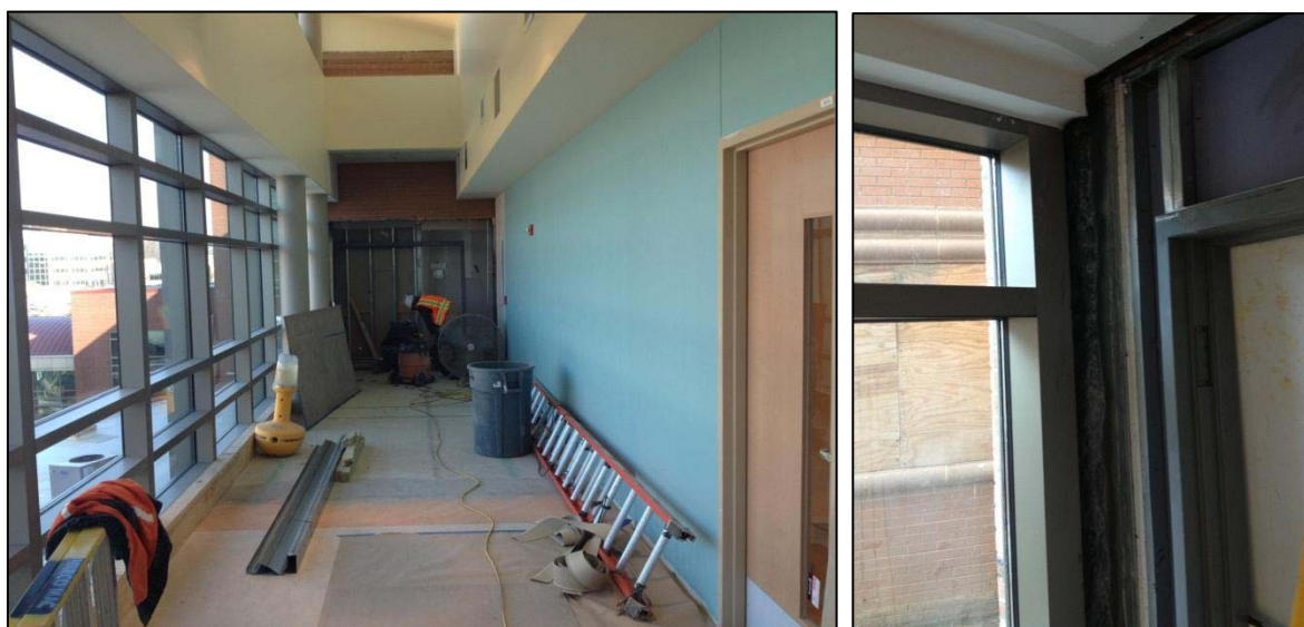
Figure 57, Left - Laborers working on the expansion joint between the floor slabs of the existing floor slab and addition. Issues required this scope of work to take much longer than anticipated due to the slabs not lining up as intended. Right - Building connection between the addition's aluminum curtain wall and existing building. Framing and a door frame can be seen already in place.
