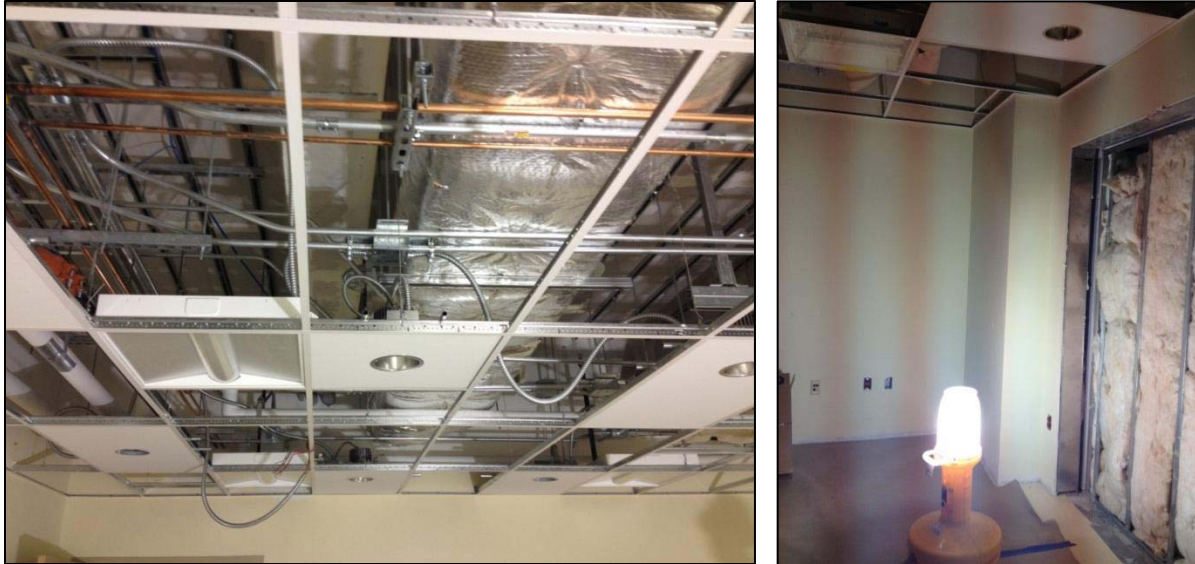
Figure 25 - Images of the CT Imaging room ceiling and temporary light fixture used inside the space. This picture was taken after a ceiling close-in inspection was performed and approved. An issue with the lead-lining required all utilities and the ceiling overhead in this room to be removed. Personal photographs taken by Chris Pozza.
